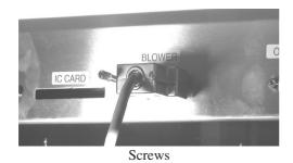
Insert one end of the signal wire cable for the blower into the connector of the electrical box.
